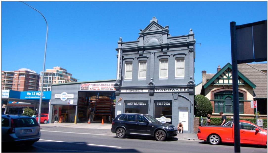
Photo 22: Photo of No. 45 Oxford Street which is a residential building currently occupied as a commercial premise (right) and Nos. 47-51 Oxford which is a two storey shop top building which is currently occupied as a retail premise by 'Bondi Junction Timber and Hardware' and has been adapted according to the needs of this business including a drive in storage and loading facility (centre). The use of these buildings clearly demonstrates that the Oxford Street retail strip is capable of accommodating adaptable uses, and will benefit from new development.
