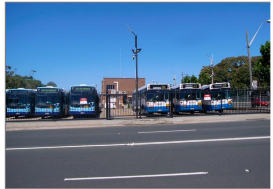
Photo 14: Photo of the bus depot as viewed from Oxford Street.
