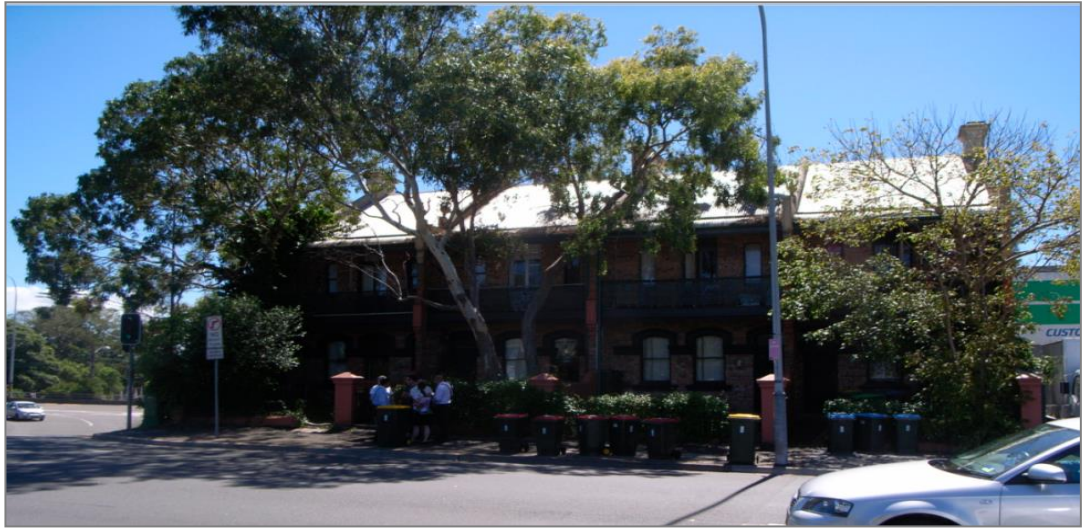
Photo 2: View of the row houses at Nos: 194-200 Oxford Street. This shows four two storey row housing with front garden areas which designate the start of the "Western Gateway" to Bondi Junction.
