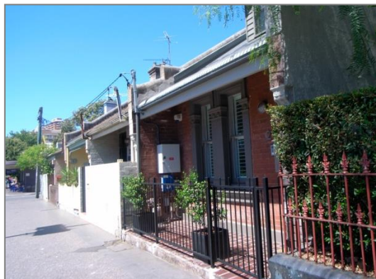
Photo 15: Photo of single storey residential dwellings located on the southern side of Oxford Street near the corner of Ruthven Street.
