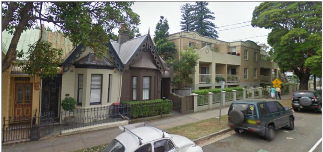
Photo 26: Image as viewed from Wallis Street demonstrating the typical dwellings and apartment buildings located on the northern side of Syd Einfeld Drive. (Source: Google)
