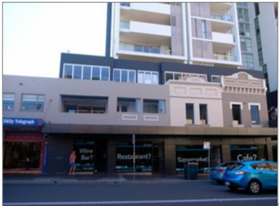
Photo 23: Photo of the mixed use development of Nos. 310-330 Oxford Street which demonstrates that the character of the existing street facades and heritage elements of the developments can successfully be integrated into the presentation of a multi-storey mixed use development.
